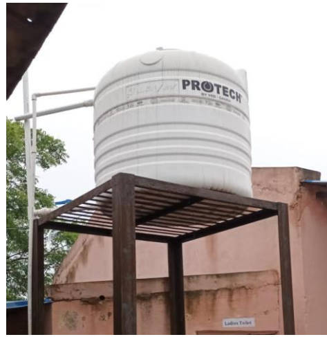
Fig No.2 Water storage
